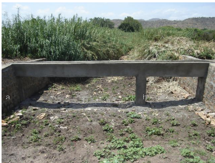
Figure 3. Irrigation canal crossing hill (a-Bakelo) and water way(b-Shewarobit)
