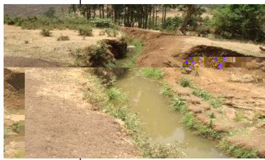
Figure 14. Unstable ditches
