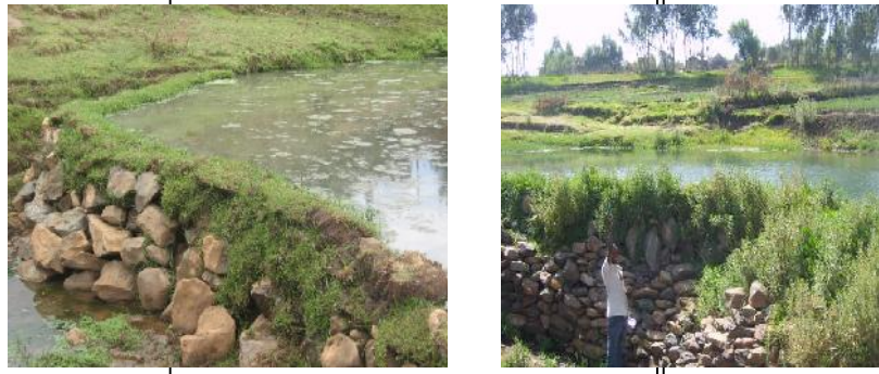
Figure 3. Diversion structure in Beles Traditional irrigation scheme
