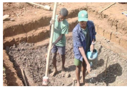
Fig. 6. Clay re-filling technique used
