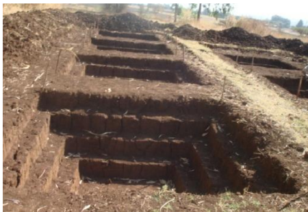
Fig.5. Step by step digging procedure
