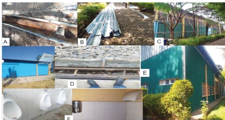
Fig. 11 A, worn-out gutter, B, New prepared gutter, C, Structure installation for gutter and workshop exterior wall maintenance, D, garage entrance construction and sliding door fitting, E Workshop and office after maintenance and F, Rest room maintenance
