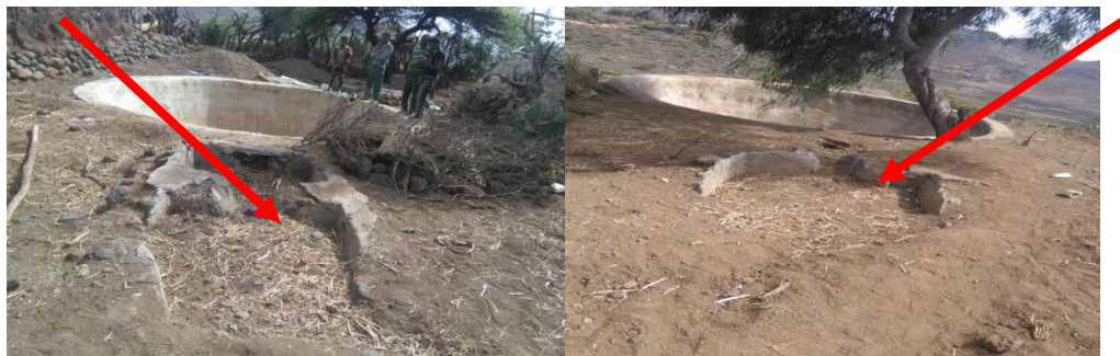
Figure 5. Silt trap full of sediments
