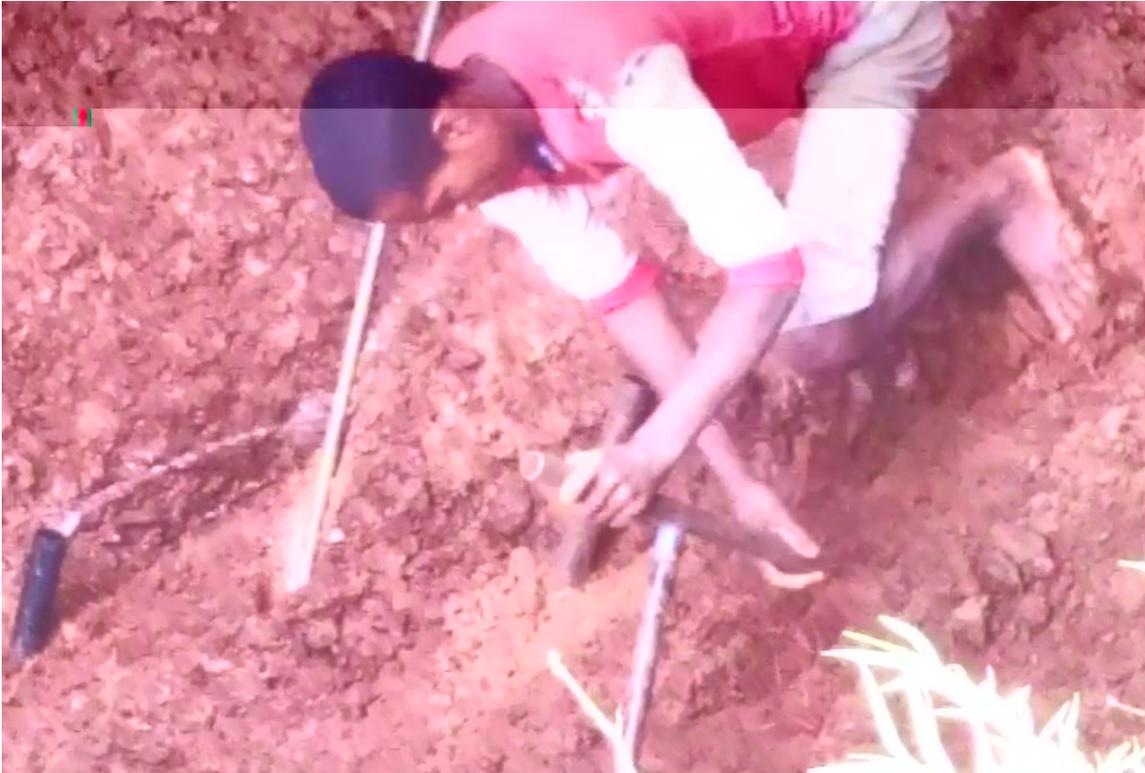
Figure 5. Observed discharges during installing the horizontal drain pipes in Vertisol gully at Debre Mawi watershed (2019). The man is installing pipes using auger of similar diameter.
