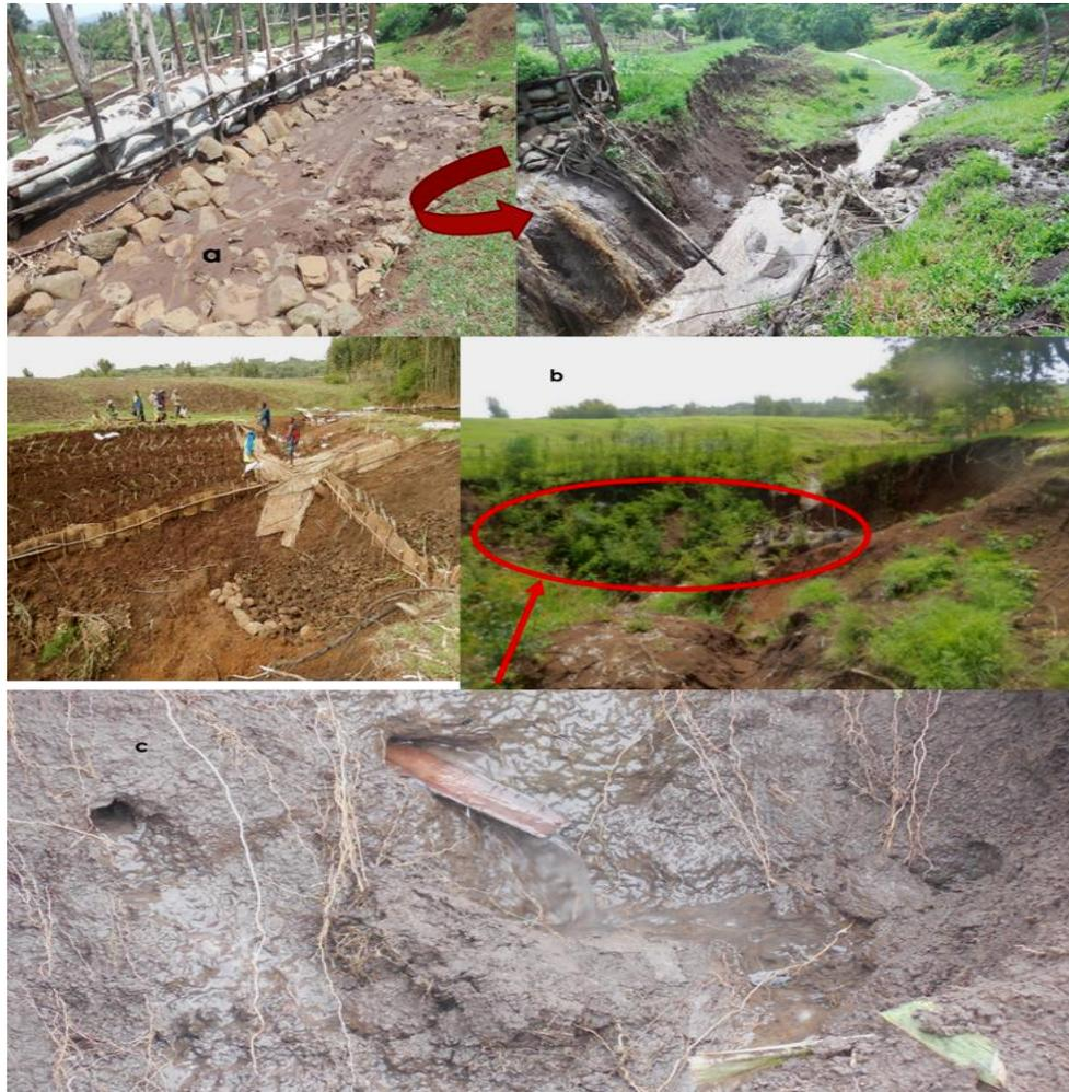
Figure 1. a) Inappropriate diversion of flowing water created another new gully, b) physical and biological headcut treatment by Zegeye *et al.* (2017) and the red circle shows the failure of planted material on the regarded bank due to wet bank, c) natural pipe dewatered the bank water and no failure was observed (Zegeye *et al.*, 2016).
